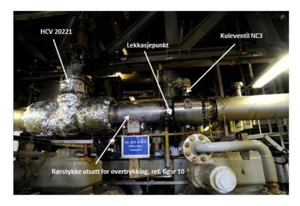
Figure 2: The pipe section between HCV 20021 and the NC3 manual shut-off valve.
