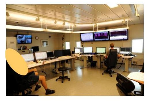
Figure 16: Shows the CCR operator at the temporary workstation as during the incident. The dedicated but inoperative workstation is to the left with a dark display.
