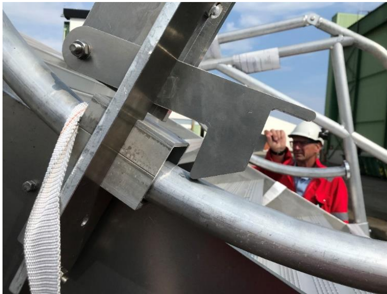
Figure 19: SS bolts washer connected directly to aluminium.
