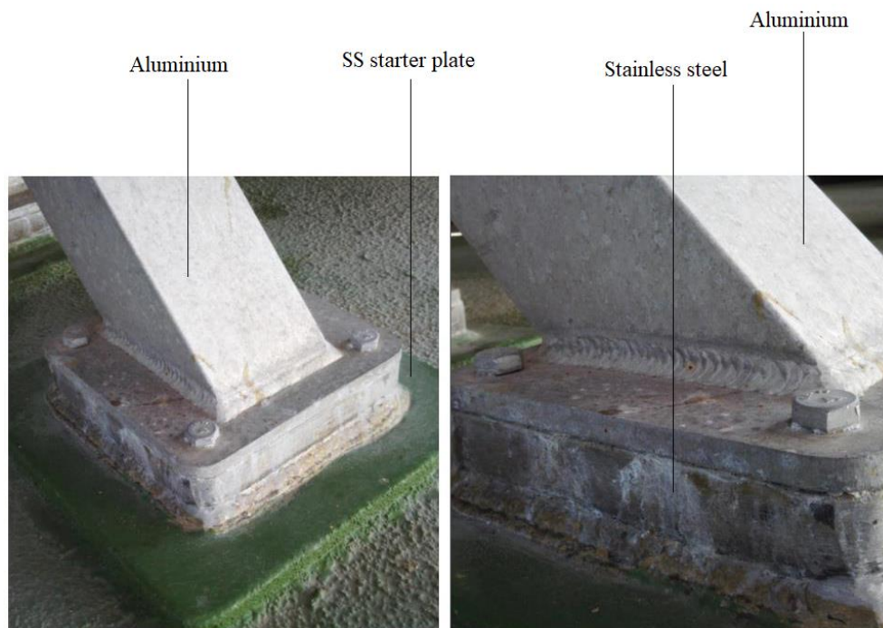
Figure 16: Corrosion in stair and access platform.
